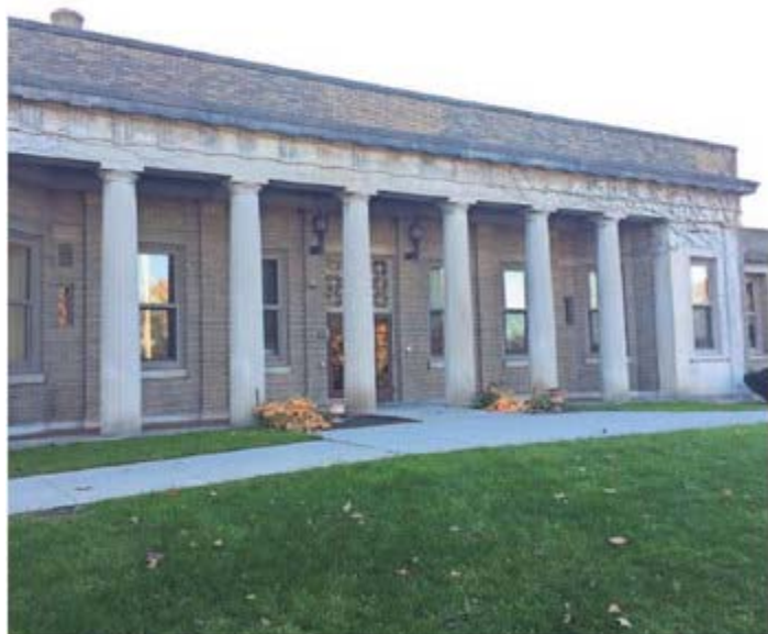
The Martin B. Anderson School 1 building on Hillside Avenue in Rochester.
