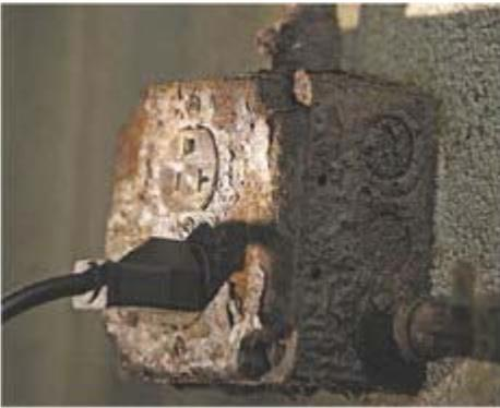
**Corrosion eats away at this electric socket and other metal pipes in the utility area near the swimming pool inside Brockport High School. JAMIE GERMANO/ STAFF PHOTOGRAPHER**
